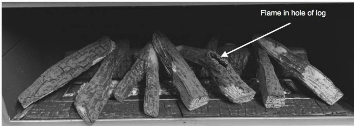
Logs positioned as above with extra Chipping's placed to suit on front fibre base
