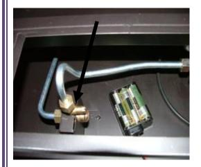
You can now decide where to route your gas pipe, knock out holes are provided in the rear and side of the fire box for use where concealed pipe work is required.
