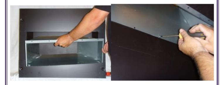
When fitting the **Liberty 6 appliance only** without the use of a chimney liner then the spigot plate must be fitted, no plate is required with the Liberty 10 model.
