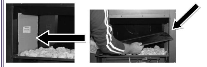
Then pass the plate through the fire opening taking care not to damage the firebox and pass through the locating slots either side of the fire outlet.
