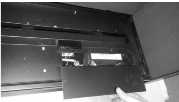
Fig 3. Remove access panel
