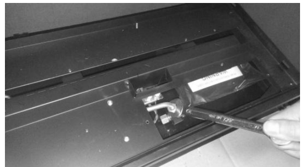
Fig 4. Disconnect gas supply pipe from the restrictor valve
