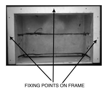
ONCE THE FRAME IS FIXED THE INSIDE OF THE FRAME MUST BE SEALED ON BOTH SIDES AND THE TOP, THE BASE MUST BE LEVELED OFF AND SEALED, MAKING THE CHAMBER FULLY SEALED AND ONLY ALLOWING THE FLUE TO PULL THROUGH THE FIRE DIVERTER AND FROM NO OTHER PLACE
