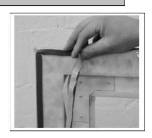
If the wall is perfectly flat it is recommended the outer frame is fitted and sealed from the inside with high temperature silicone ,fire cement or sand and cement
