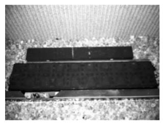
The granules can then be spread around the fire tray and behind the fibre strip packing it to ensure the strip cannot move
