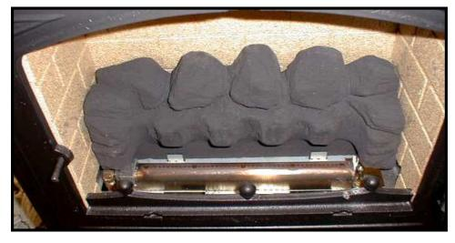
and the base of the coal locates behind the tags on the burner.
