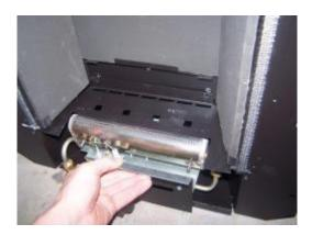
You can now place the burner tray into the firebox making sure that the fixing points are locate properly on the firebox.
