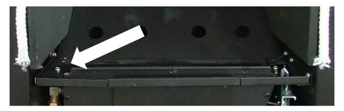
Fit the two securing screws through the front plate ensuring that the plate is in correct position in the box; secure the two screws at the back of the tray. Connect the gas supply and tighten the gas connections.
