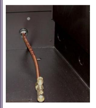
You can now decide where to route your gas pipe, knock out holes are provided in the rear and side of the fire box for use where concealed pipe work is required.
