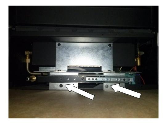
Remove the 2 screws on the top of the burner tray.
