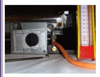
Check that the inlet gas pressure is at 20 mbar / Working Pressure at 20 Mbar (+/- 1 mbar) Light the pilot and check the correct operation of the burner at all the flame settings.
